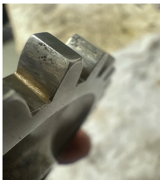
Above: It doesn't take much for corrosion to start as surface pitting on steel parts. Right: Tropic Ocean Airways is experienced in combating water and moisture.
